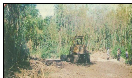
Building a road in Morobe Province
